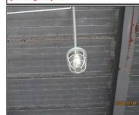
Photo of chemical storage room (if applicable) Explosion-proof light.JPG
